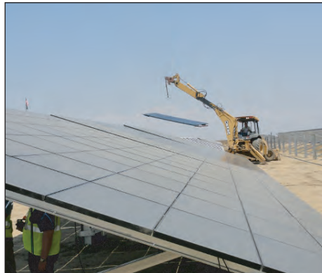
Solar Frontier's CIS PV panels being installed.
