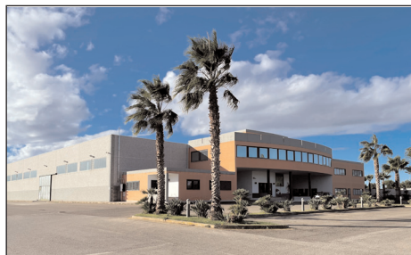
Midsummer's factory in Bari, Italy.
