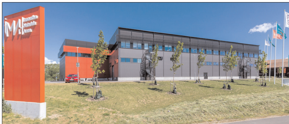
SweGaN's new headquarters and production facility in Linköping, Sweden, to be completed by the end of second-quarter 2023.
