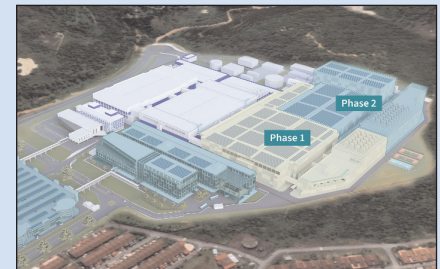
p15 Infineon is expanding its plant in Malaysia — over and above the original investment announced in February 2022 — by building the world's largest 200mm silicon carbide power fab.
