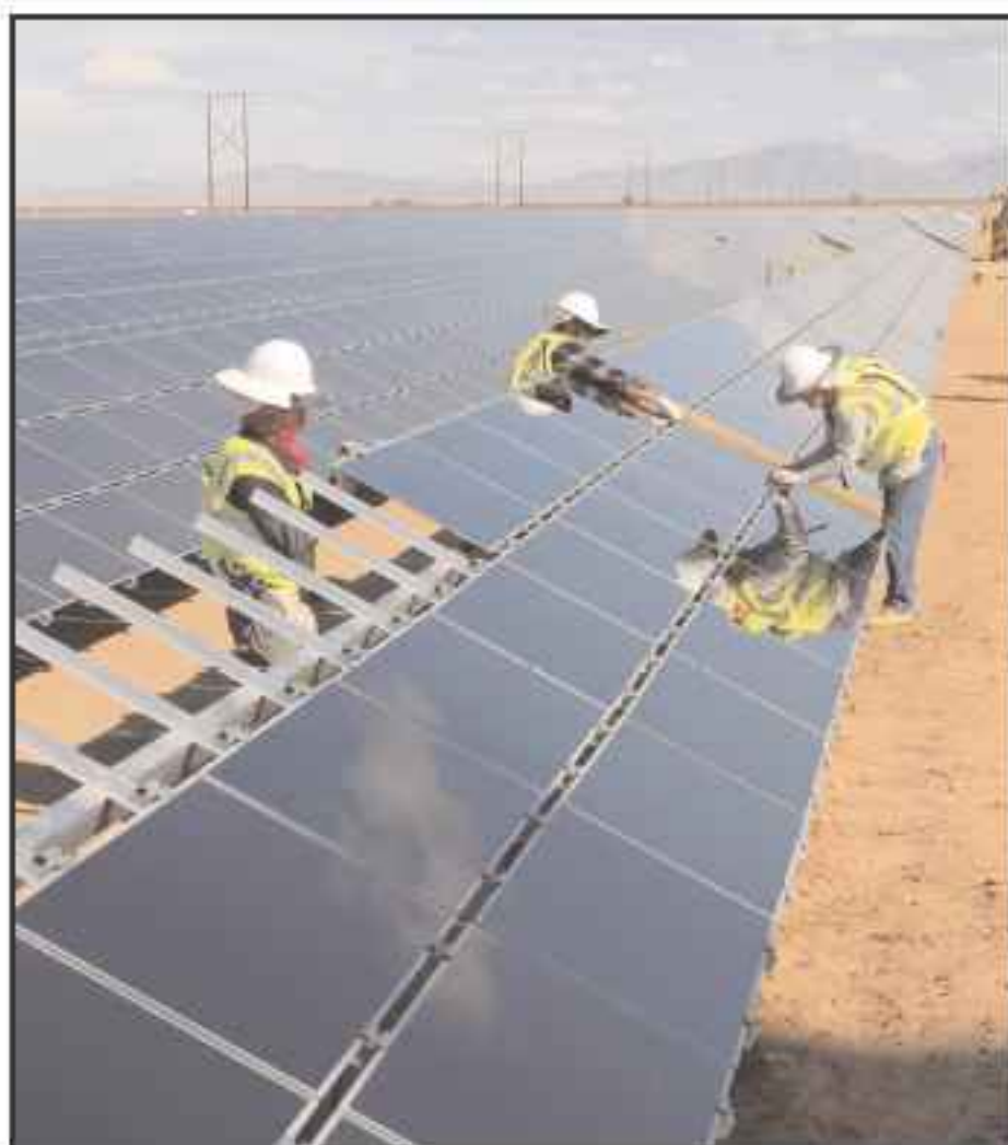
First Solar working on finishing the 21MW Blythe plant.
