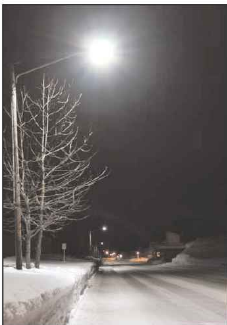
LED street lights in Valdez.
