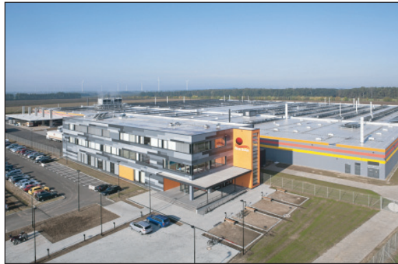
First Solar's new factory in Frankfurt (Oder), Germany, inaugurated after reaching full production in October.
