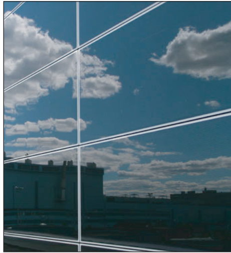
The solar panel façade is based on solar panels made from glazed PV modules and Ruukki's steel rain-screen panel system.
