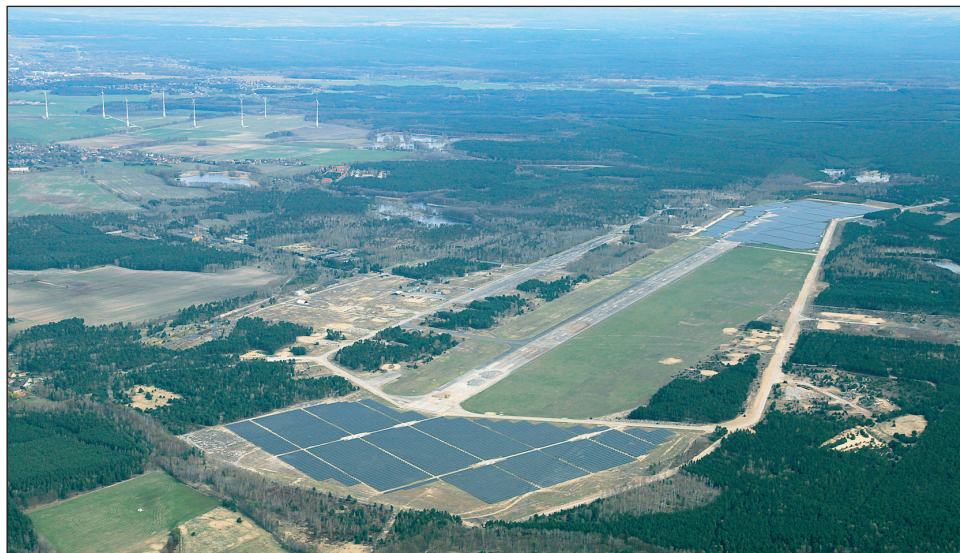
Aerial view of Jocksdorf and Preschen solar parks. Source: Phoenix Solar.
