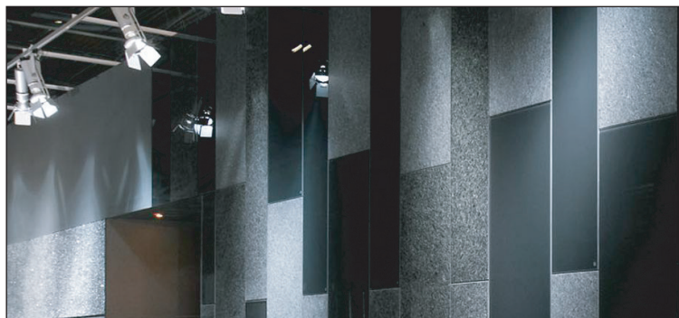
Solar façades using building-integrated photovoltaics.
